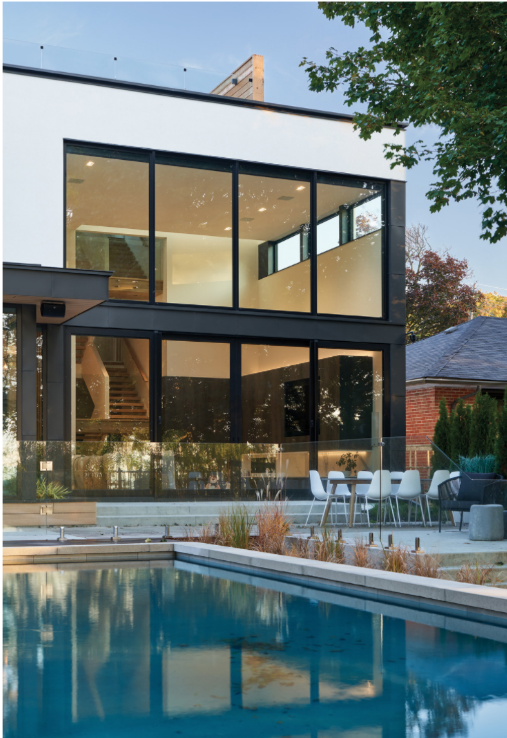
The house embraces the landscape – large sliding doors open out to the backyard and pool, and an exterior planter reappears inside between the great room and dining room. Photo credit: Doublespace Photography Inc.
